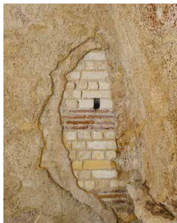
5 Superimposition of plaster layers
